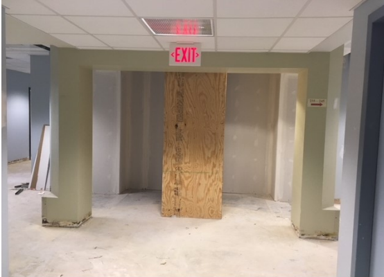
The Ben statue is protected with a plywood box during construction.
